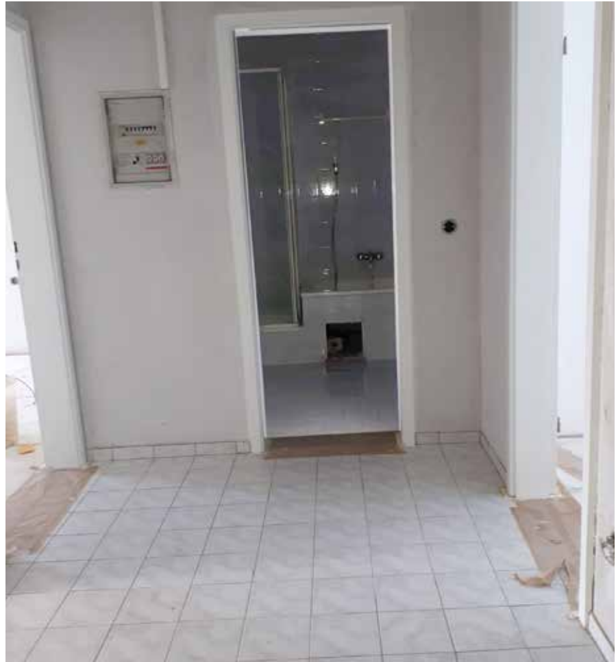
Blick in den Flur
